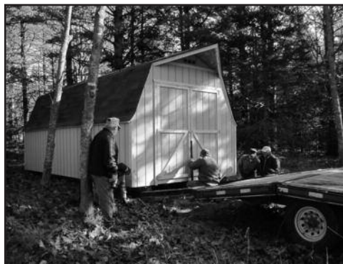
Club members off-load the new equipment storage shed near the clubhouse and picnic grove.
