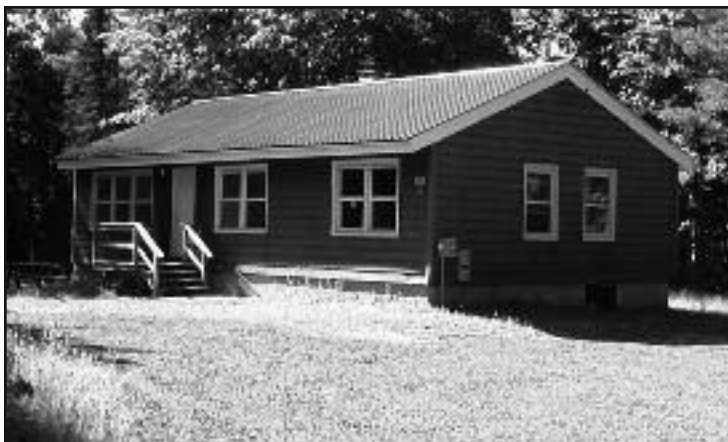
CKSC Phoenix Farms clubhouse sports a new green metal roof and other improvements completed by member volunteers. Thanks to all who donated their time!
